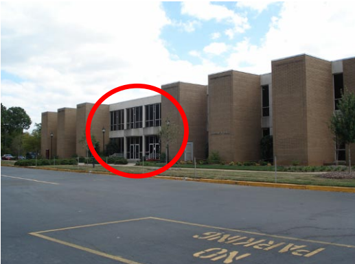
Hubbard Hall: potential signage location
