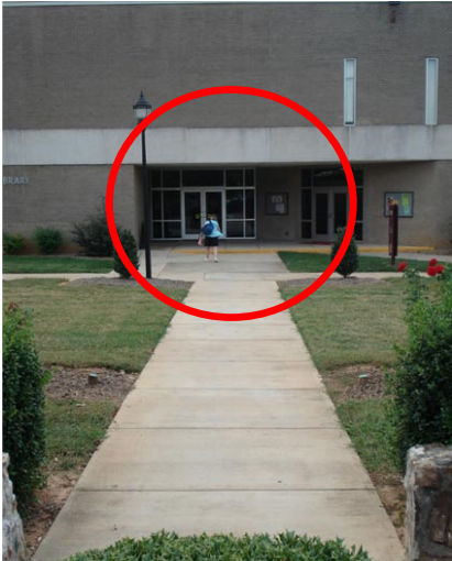
Signage, landscaping and lighting can create a more welcoming entrance into the Medford Library.
